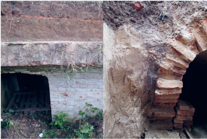
Left: Individual layers of backfill above the vault of the main gallery in front of bastion No. 4 during the 2016 repairs. Right: The visible distinction between the original ground level and the subsequent backfill of a level 1 mine branches in front of ravelin No. 18. (Jiří Hofman).
