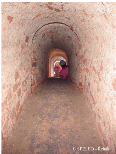
View of the inclined section of the level 1 mine branches featuring slots for timber beam insertion. (SPELEO – Řehák).
