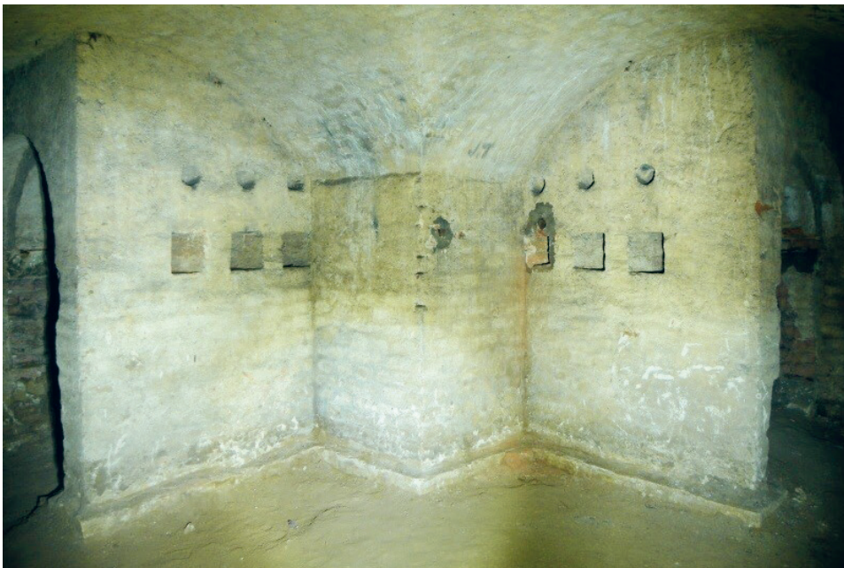
Interior view of the tambours featuring traverses and entrances to the envelope. (R. Gazsi).
