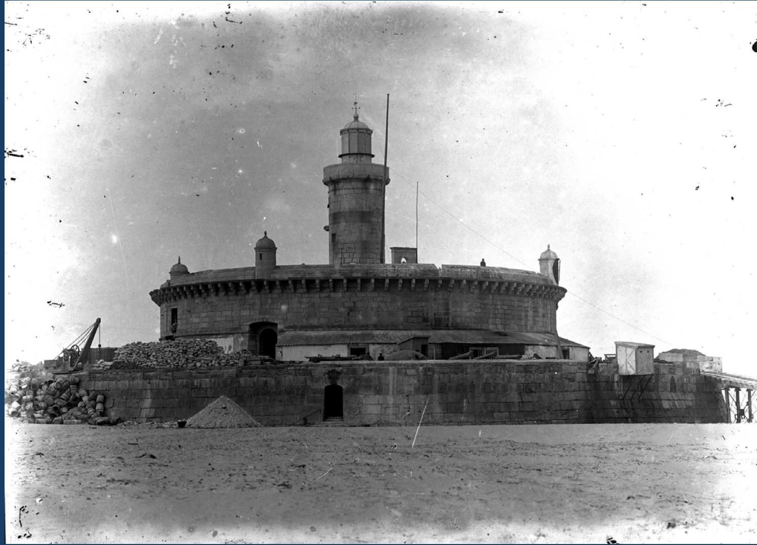
Bugio Fort, maintenance works, 1930-1932, photo by Alberto Carlos Lima, in AFCML, Photographic Archives of Lisbon Municipality.
